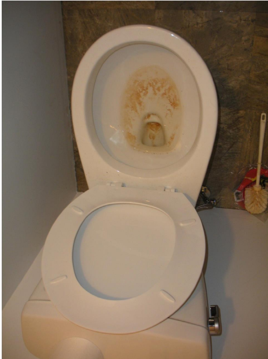
Figure 4 - Staining of toilet from high iron in well water
