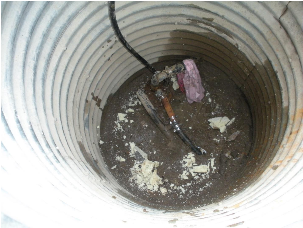
Figure 5 - Leaking well seal in a well pit
