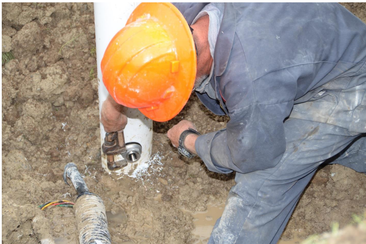
Figure 6 - New PVC well casing used to extend well casing above ground and new pit-less adapter installed
