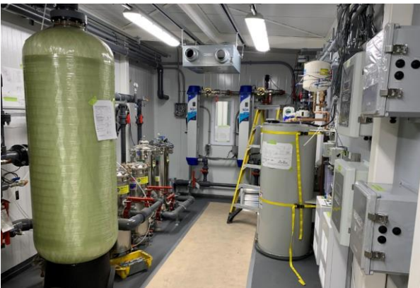
Pictured: UV equipment inside the water plant
